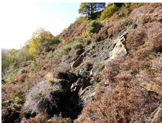
Figure 11: Tension cracks above Pantteg Chapel
