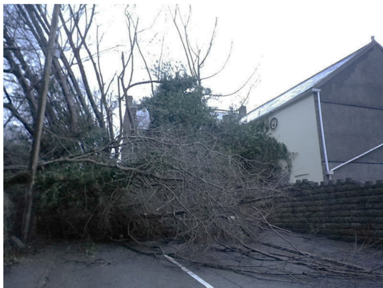
Figure 8: Landslip at Pantteg Chapel, December 2012, (Website accessed November 2015)
