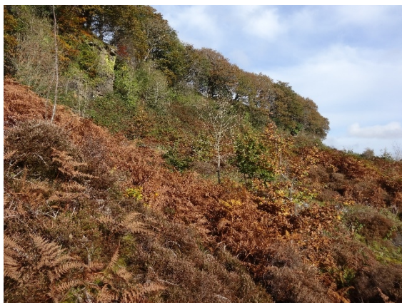
Figure 9: Landslip backscarps above Pantteg Chapel
