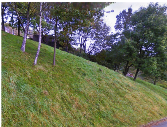
Figure 10: Landslip lobes along Clees Lane
